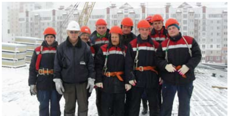
Foreman Viktor Zukov with builders in the construction place of supermarket "Oma", Minsk (Belorussia)
