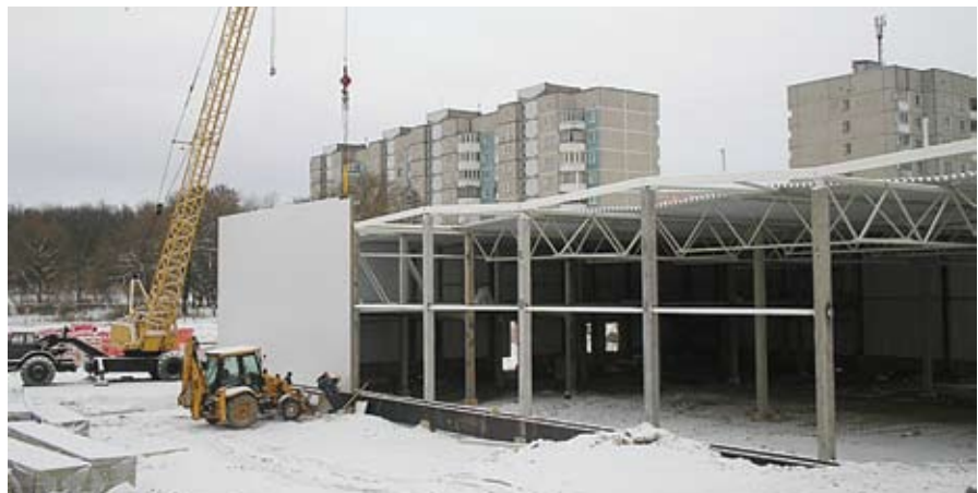
Construction of a supermarket in Grodno (The Republic of Belarus).
