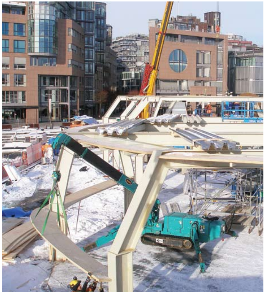
Construction of a restaurant in Oslo center (Norway).
