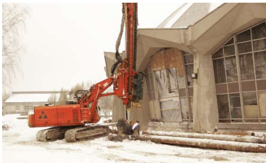
Reconstruction of the ice arena in Elektrėnai (Lithuania).
