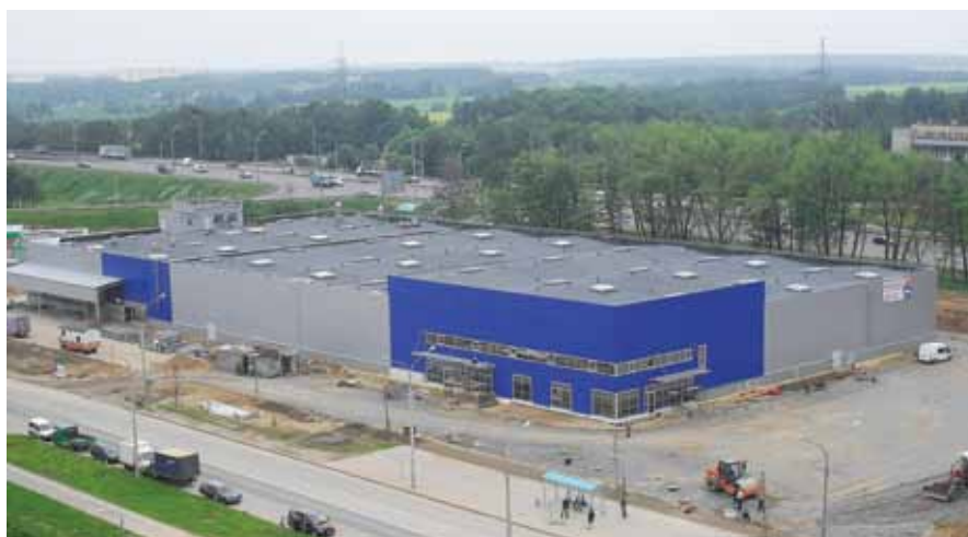
Construction works of the supermarket in Minsk (Republic of Belarus).
