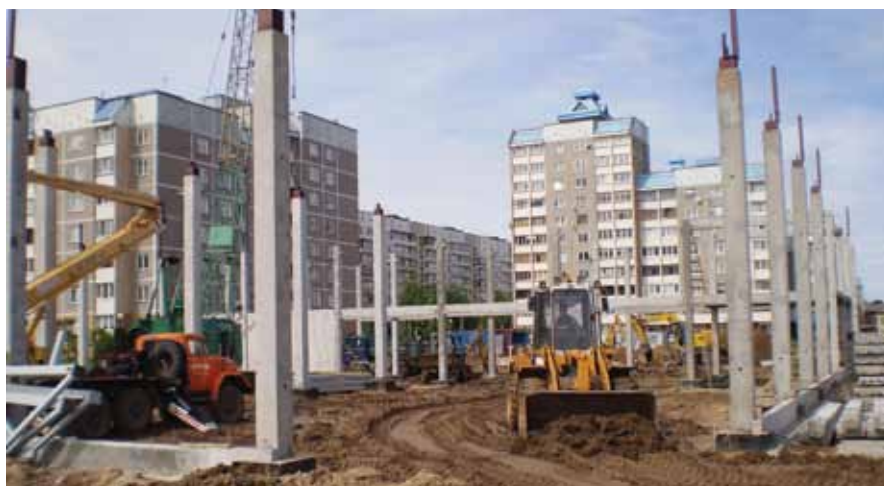
Construction works of the supermarket in Grodno (Republic of Belarus).
