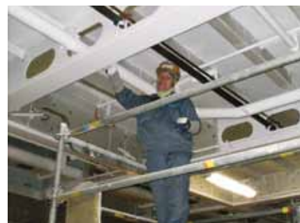
Insulation works (Finland).
